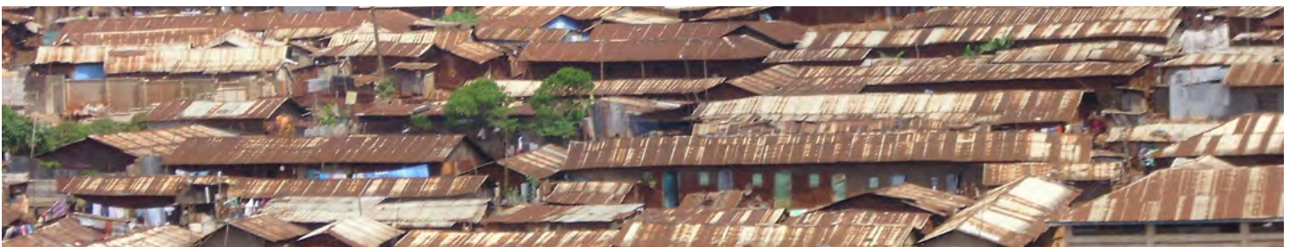
Structures in Kibera. < http://affordablehousinginstitute.org >
